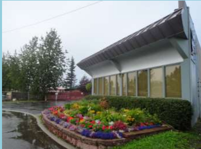
Anchorage Office- Photo courtesy of Adak Eagle Enterprises
